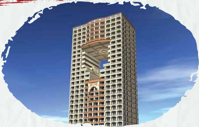
Digar Al Bahr Tower
