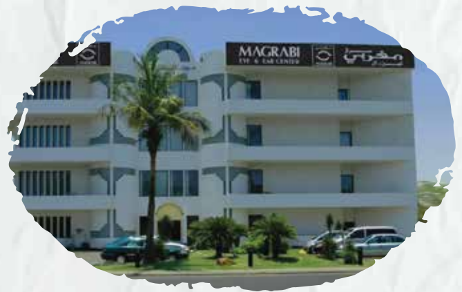
Magrabi Optical Co. (Maintenance of firefighting systems and early warning systems against fire risks).
